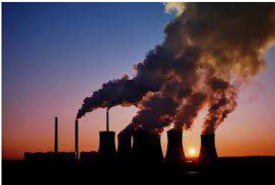
Smoke emission from chimneys
